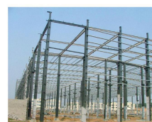
钢结构工程 Steel structure engineering
